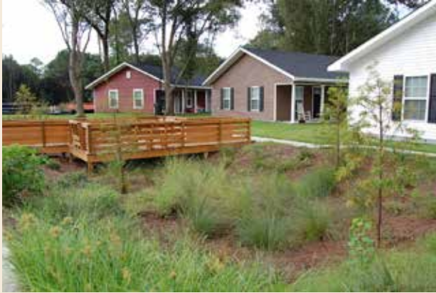
Central bioretention basin serves a dual purpose for community open space and stormwater treatment.
