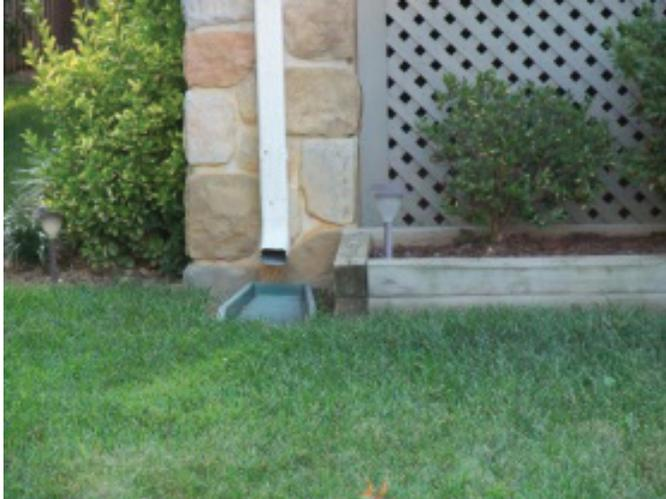
Figure 4.7-1. Simple Rooftop Disconnection
